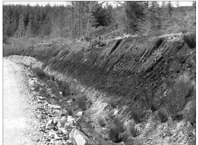
Access road cut through peat over three metres deep for timber extraction and access to windfarm. Trees growing on peat have poor stability and are easily windthrown as above when operations like road building or clear felling expose them.
